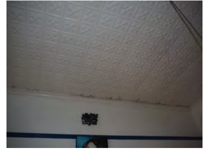
Figure 2. 83: Pressed metal ceiling to front bedroom.
