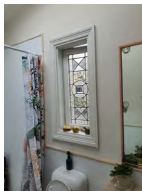
Figure 2. 156: Leadlight glazing to bathroom window.
