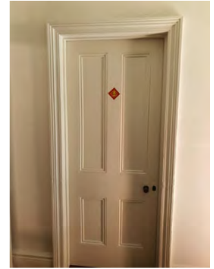
Figure 2. 132: Typical internal four panelled door.
