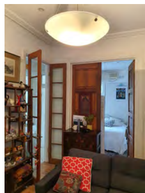
Figure 2. 155: Later French doors and enlarged door opening.
