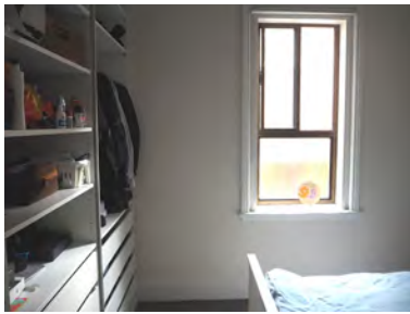
Figure 2. 70: Front bedroom with original window architrave and later aluminium framed window.
