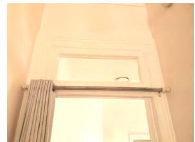
Figure 2. 102: Typical door architrave with fanlight.
