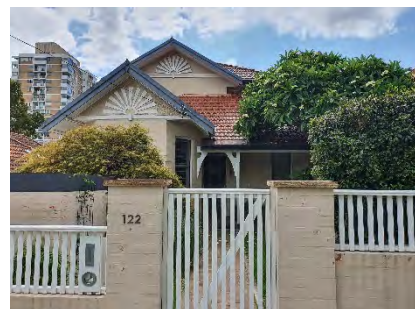
Figure 3. 8: No. 122 Benelong Road with rising sun motif to front gable. The gable located behind appears to be a later addition, also with a rising sun motif.
