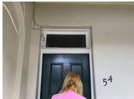
Figure 2. 28: Front door with fanlight and dentil mouldings matching those at No. 50 Parraween Street
