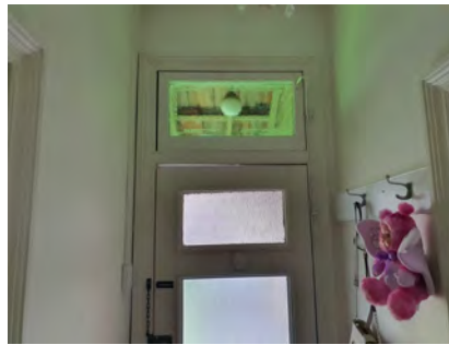
Figure 2. 140: Coloured glazing to front door fanlight.
